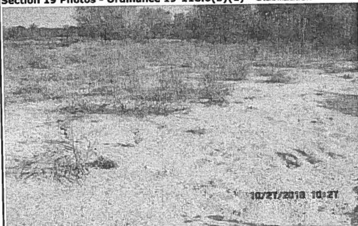
The site is loose soils from former construction activity. Overdue to be made permanently stable.
